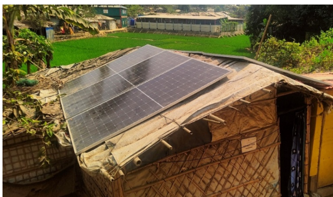
Photo 8: Installed 3kWp solar PV panels on a shelter roof in the Refugee camp ©IUCN
