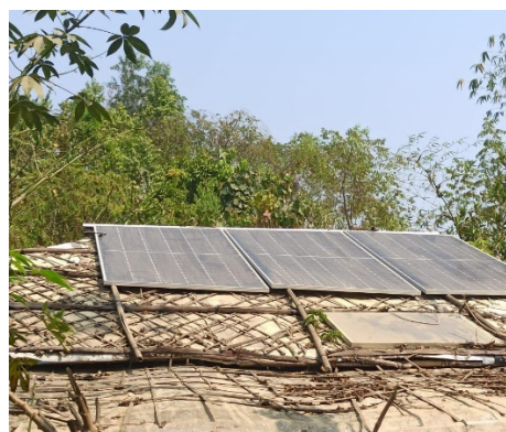
Dust accumulation on solar panels just two days after installation ©IUCN
