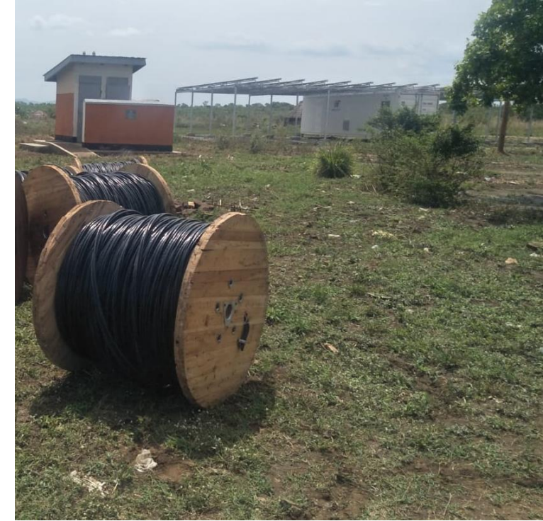
Mini-grid site outside Palabek settlement.
