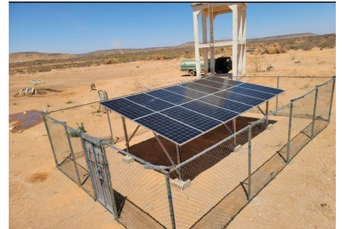
Water pumping in Kismayo © RDI
